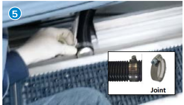
Tighten the hose with joint.
