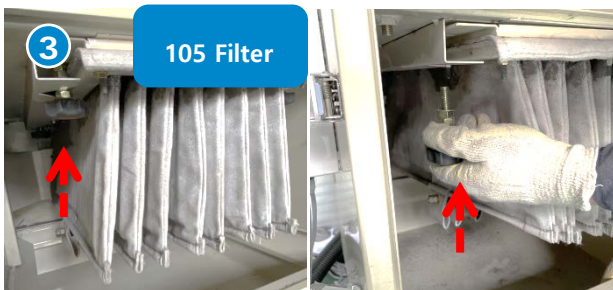
Loosen the four edge fixing screws.
