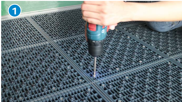
Loosen volts in the Modular Cell with Cross(+) Screw Driver.
