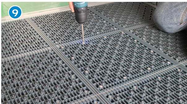
Tighten the bolts again.
