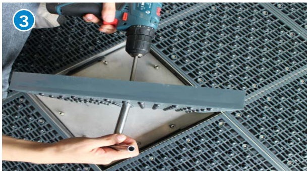
Fix the Pin with Zig, and loosen it with Cross(+) Screw Driver.
